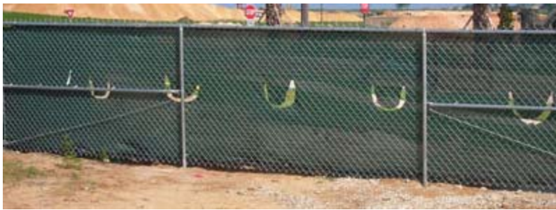
Construction LOD Fence
